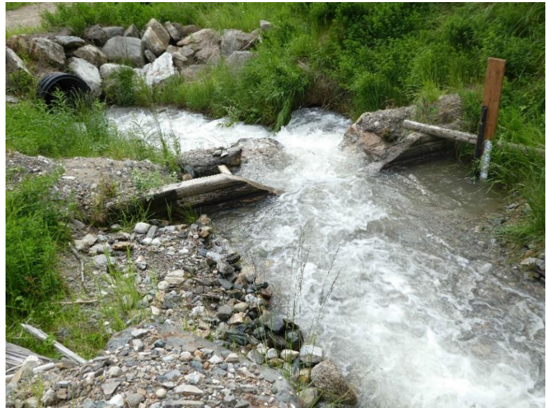
b) Gar station – staff gauge and weir
